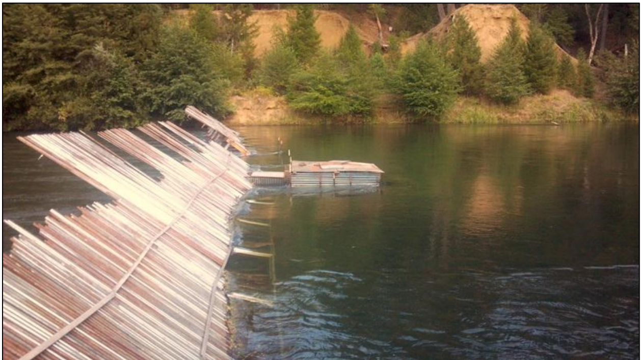
Figure 3. Set up of Junction City weir (JCW), 2015. Note single trap box with boat gate just beyond.
