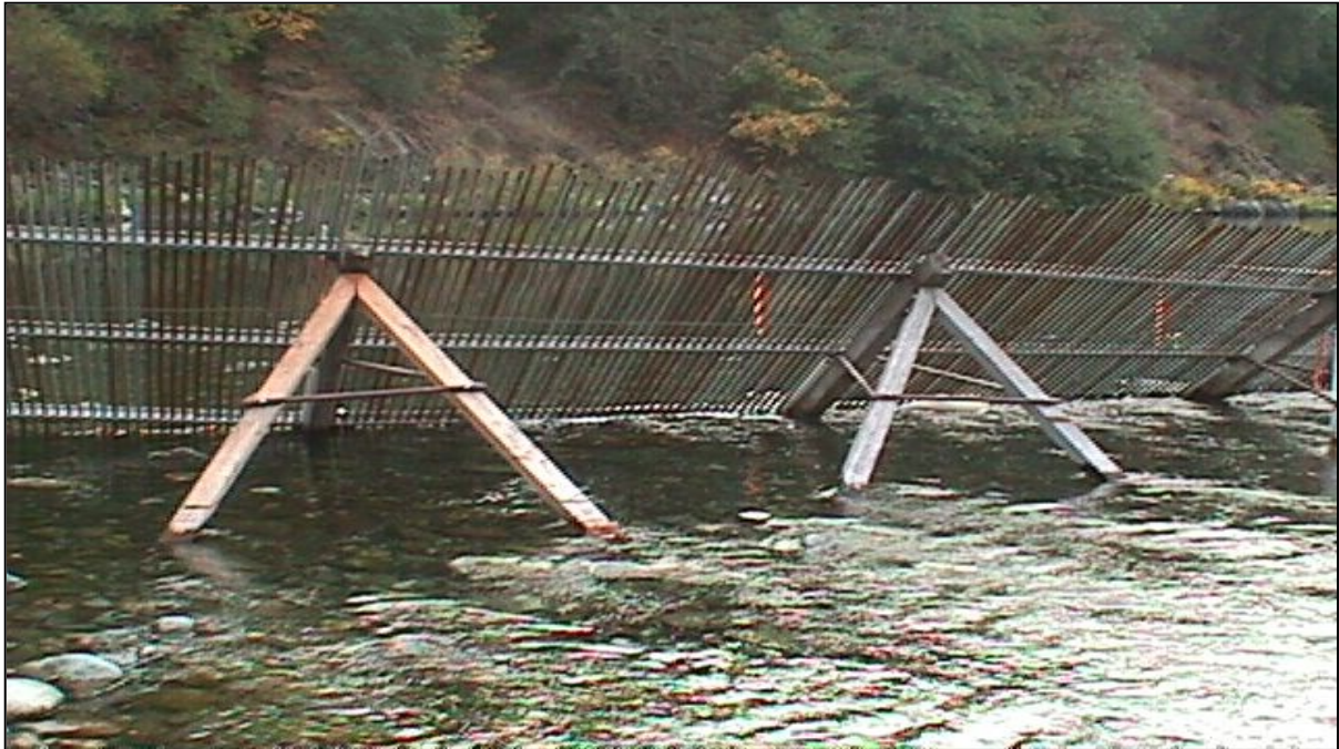
Figure 2. Photograph of Alaskan-style weir, tripods, support channels, and conduit (looking upstream). Picture taken at Willow Creek weir, 2015.
