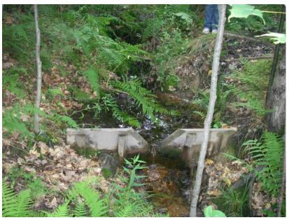
For use on small stream channels with depth where other methods are not feasible, or a high degree of accuracy is required (Flow studies).
