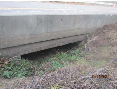
Figure 11. Sediment accumulation in culvert at MRN 1 27.92. Downstream looking upstream. November 2014.
