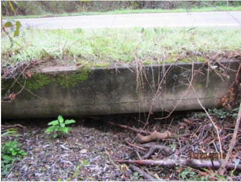
Figure 10. Sediment accumulation in culvert at MRN 1 14.86. Upstream looking downstream. November 2014.
