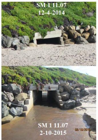
Figure 26. Comparison of highly variable sediment conditions at SM 1 11.07.
