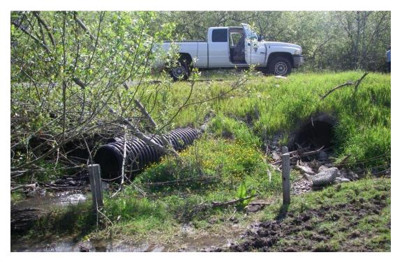
**Figure 3.** Driveway stream crossing (Culvert #3) containing four separate culverts on the Unnamed Tributary to the Smith River. All three culverts are temporal upstream barriers to juvenile salmonids.
