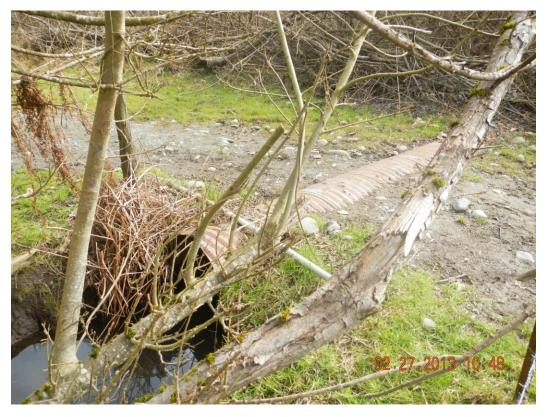
**Figure 4.** Livestock culvert crossing (Culvert #2). The culvert is undersized and the inlet was plugged with woody debris at the time of the survey.
