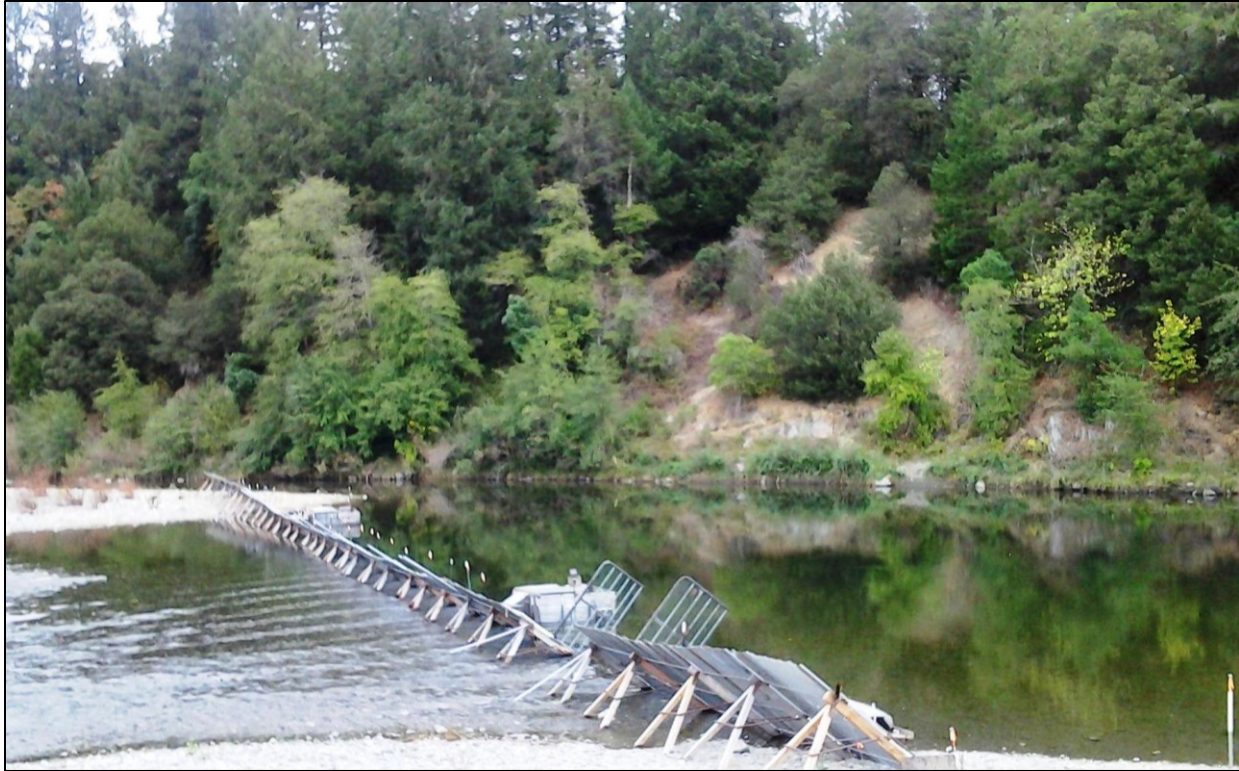
Figure 4. Picture of standard Willow Creek weir (WCW) configuration, with two trap boxes.
