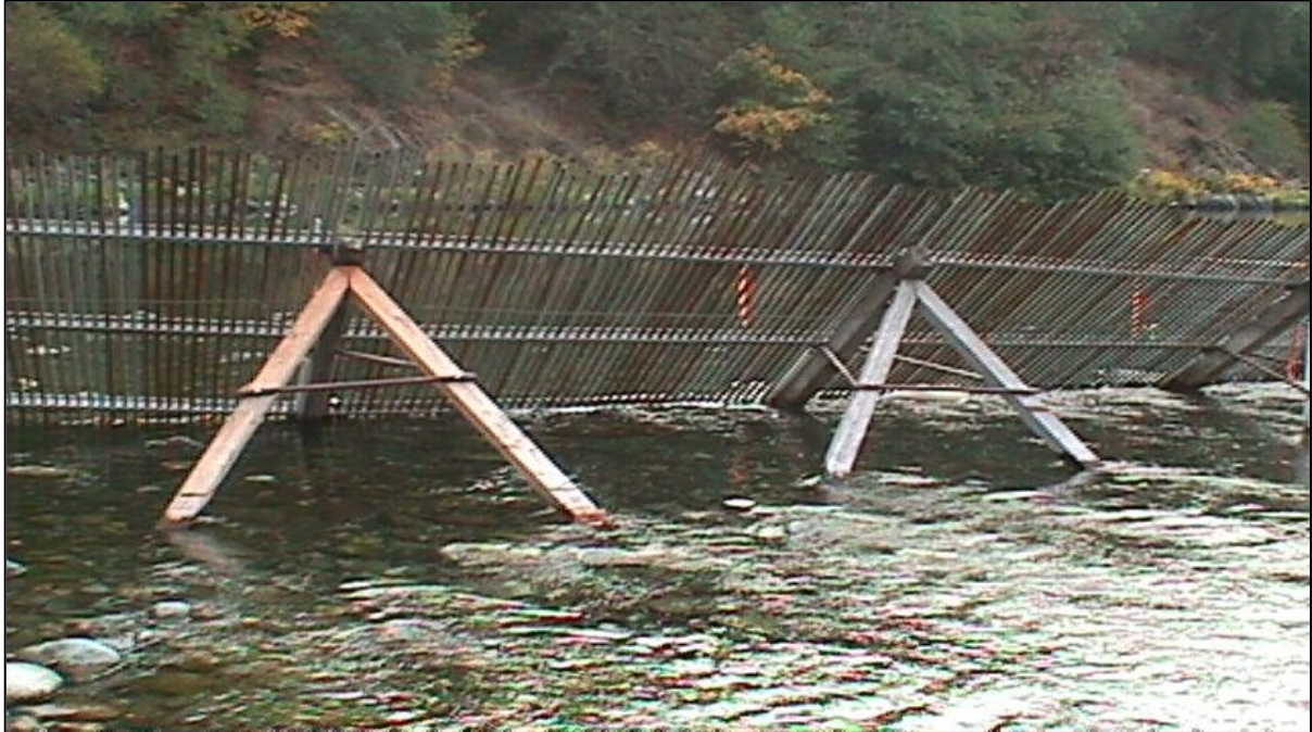
Figure 2. Photograph of Alaskan-style weir, tripods, support channels, and conduit (looking upstream). Picture taken at Willow Creek weir, 2016.
