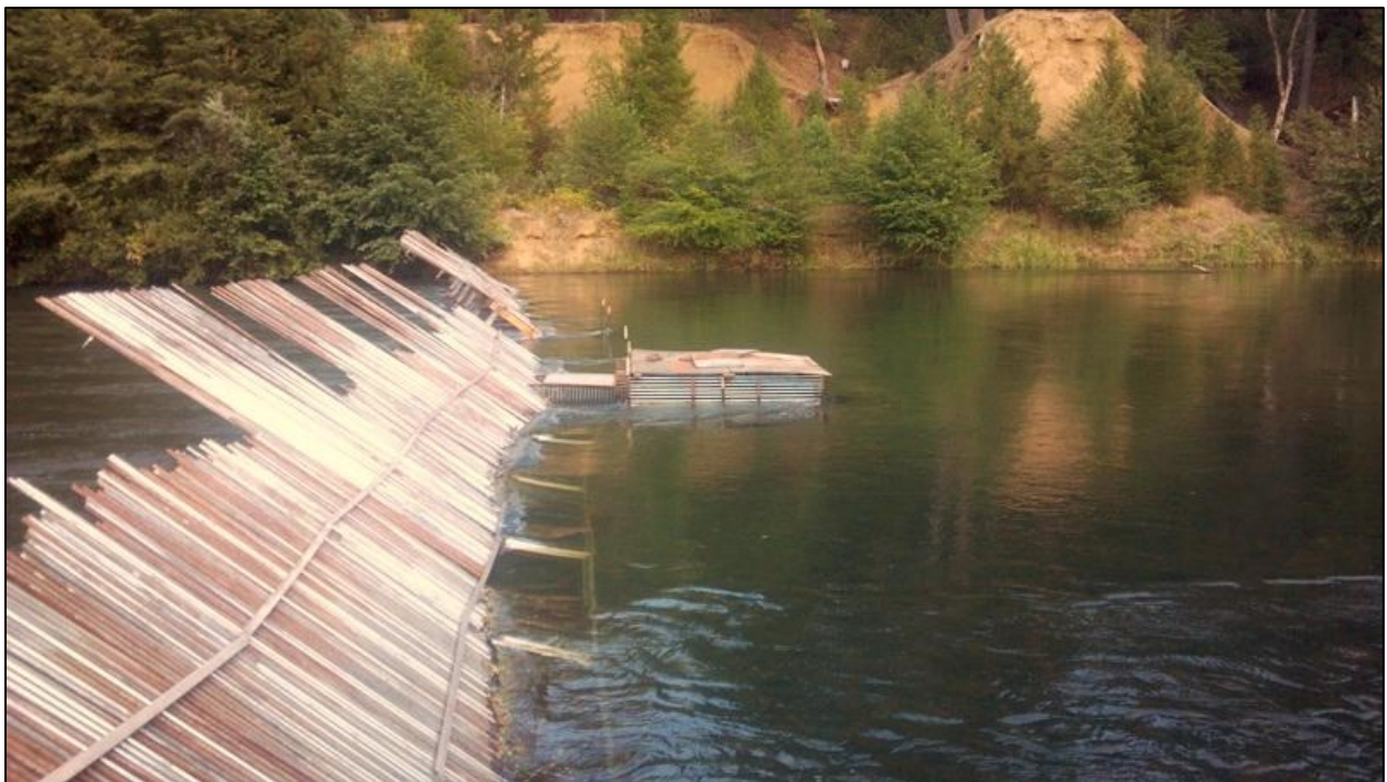
Figure 3. Photograph of Junction City weir (JCW) in configuration used in 2016. Note single trap box with boat gate just beyond.
