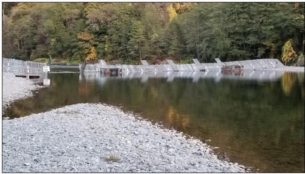
Figure 4. Willow Creek weir in 2020 (in "open" mode), with standard boat gate and two traps. Flow is from right to left.
