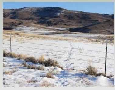
Tracks reveal where mule deer now easily cross Eastfork Livestock's new wildlife friendly fence. Twelve inches between the top two wires, a smooth bottom wire placed at least 16" high, and a top wire no more than 42" high make a friendly fence.
