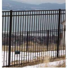
Above: A solid top rail and narrow vertical bars on this iron fence reduce hazards to wildlife.
