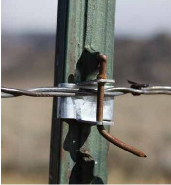
Existing fences can be readily modified by installing staple locks to create a drop wire so wire height can be adjusted when livestock are not present.
