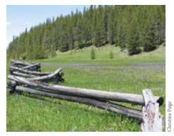
A low worm fence is easily hopped by most ungulates. Drop the top rail to the ground every few hundred feet to allow smaller animals cross.
