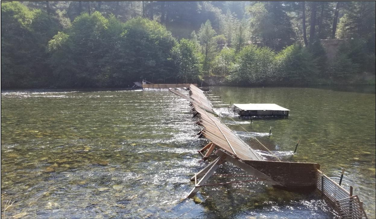
Figure 3. Junction City weir (JCW) configuration in 2018 after the JW 30 rebuild. This shows the weir in trapping mode. Stream flow is right to left.
