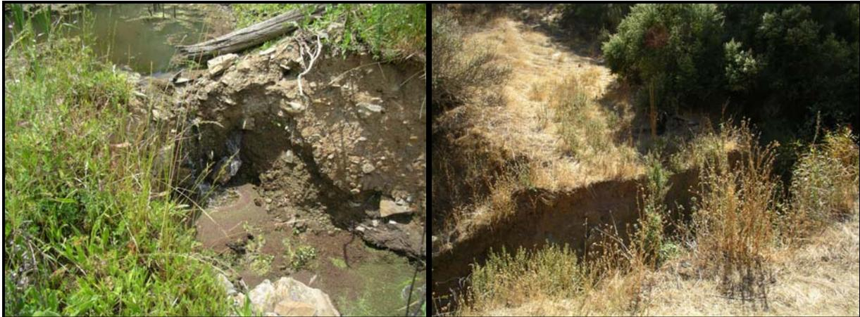
Figure 7. San Luis Reservoir Wildlife Area firebreak at Lost Pond during early stages of erosion (at left, 2005) and after completely washed out with pond no longer dammed (at right, 2006).
