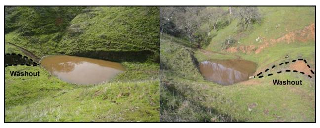
Figure 3. Upper Cottonwood Creek Wildlife Area berm erosion at Big Bully Gully while viewing pond from east side (at left) and from southwestern side (at right), 2006.
