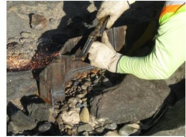
Figure 1: Cutting Low Flow Notch
