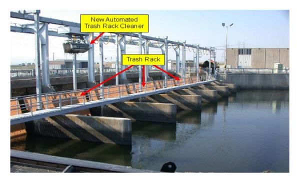
Figure 5. View of the new SDFPF trash rack and automated cleaner.
