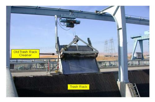
Figure 11. View of the old trash rack cleaner and old trash rack.
