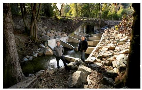
Figure 5-1. Example pool-weir fish ladder designed to improve salmon passage, but not well designed for Pacific lamprey passage. Source: <u>http://www.pressdemocrat.com/article/20140109/articles/140109595</u>
