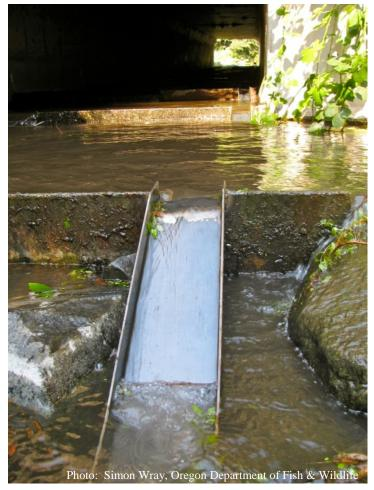
Figure 5-2. Example of installation of lamprey ramps to improve passage in Threemile Creek, Oregon.
